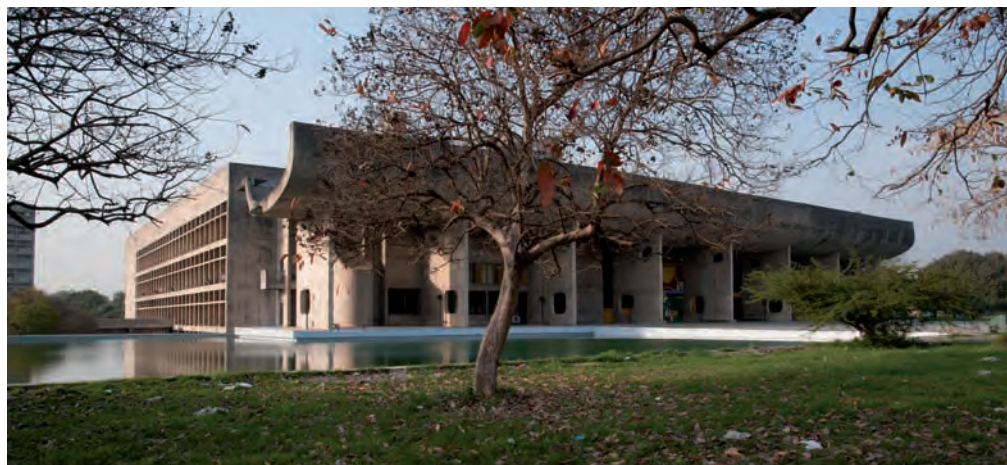
Fig. 1 Palace of Assembly in Chandigarh's Capitol Complex designed by Le Corbusier, 1951-1963 (photograph: Franco Panzini)
